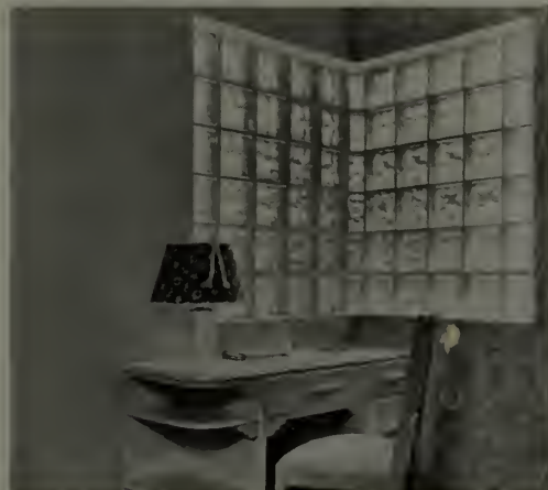
SHUT OFF THAT UNATTRACTIVE VIEW with PC Glass Blocks . . . and you won't have to sacrifice daylight. A smart corner panel provides light from two directions, makes the room more comfortable, and easier to heat, because PC Blocks have high insulating value. J. F. McKeage residence, St. Petersburg, Fla.
